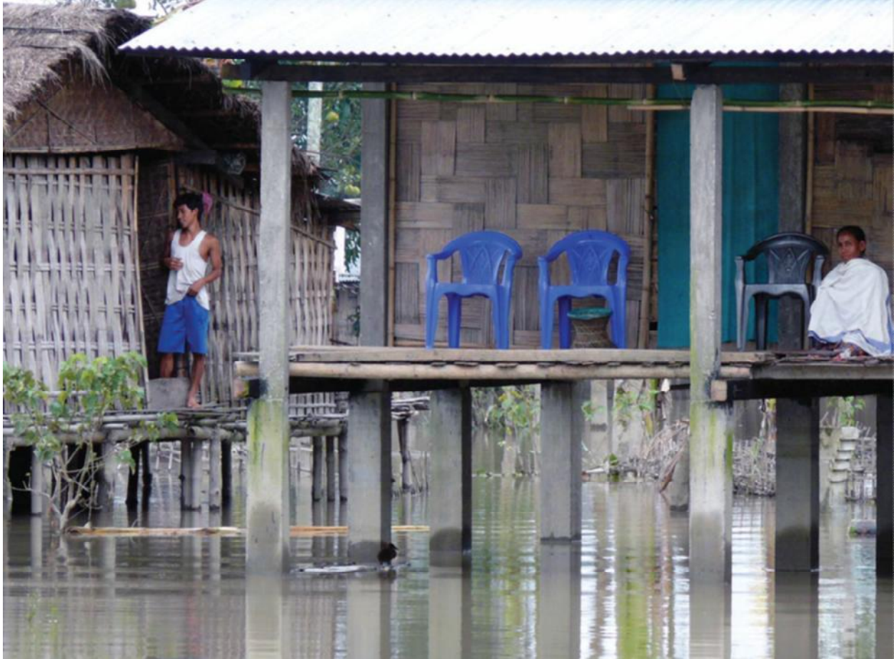
Two types of chang-ghar (house on stilts of the Mishing community): left, the original design of bamboo and wood; right, wealthier households invest in concrete to make higher stilts
