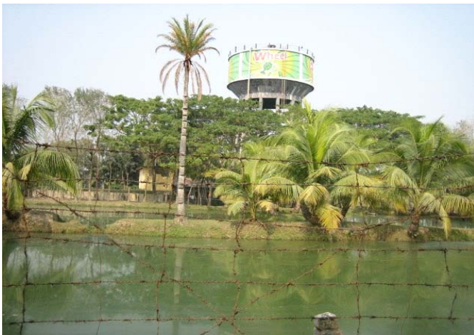
Urban water supply
